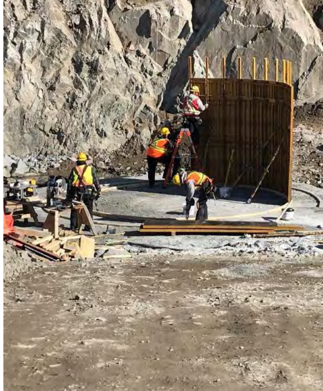
Timmiak Construction Limited employees construct a raise bore collar for the Vale underground mine. The collars will lead to shafts that allow fresh air to be pumped in and stale air to be pumped out. A fifth shaft will provide an escape route for underground miners. Photo: Timmiak Construction Limited
